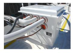
Is a contractor constructed "doghouse" tested to ASTM-E-2357-11 standards? This calls for a minimum of 75pa to pass an air permeance test by a third-party certified lab. The  $\underline{\text{VAULT}}$ ® surpassed 300pa and is warranted for 20 years.
